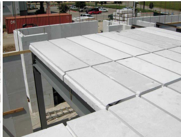
Figure - 9. Typical side bearing detail of slabs panel.
