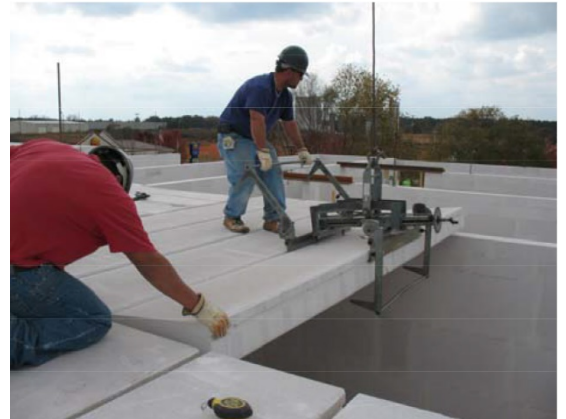
Figure - 5. Before placing the panel on the supports, clear safety bar from adjacent panel.
