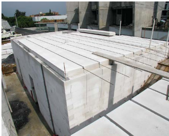
Figure - 8. Typical detail of panels supported on ASLAN AAC Wall.
