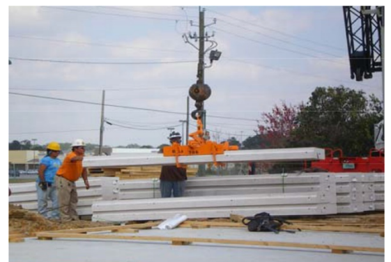
Figure - 4. Placing the lifting gear at the center of panel.
